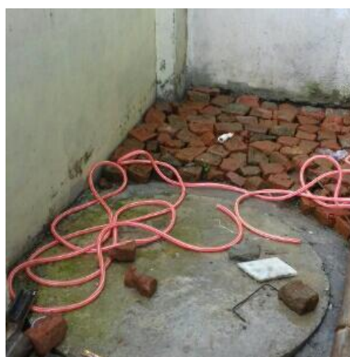
Figure 2: Containment system (HHs Survey, 2019).
