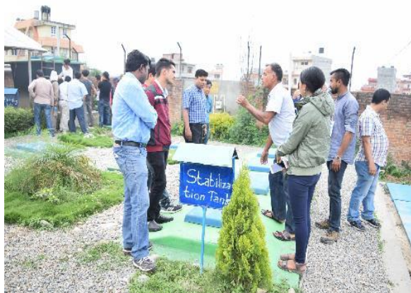
Fig-17: Mr. Surya Prasad Ghimire, caretaker of FSTP, Lubhu explaining about stabilization tank of treatment plant.
