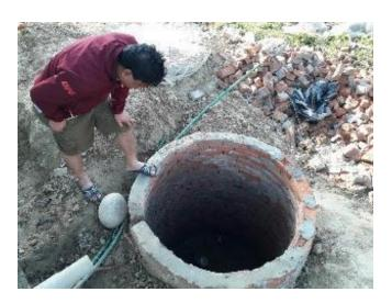
Figure 8: A soak pit constructed to discharge effluents.
