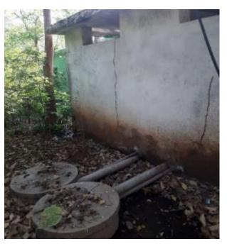
Figure 9: Toilet connected to lined pits.
