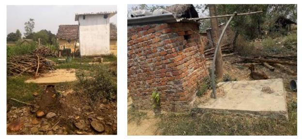
Figure 8: Toilet connected to biogas digester and a fully lined tank.
