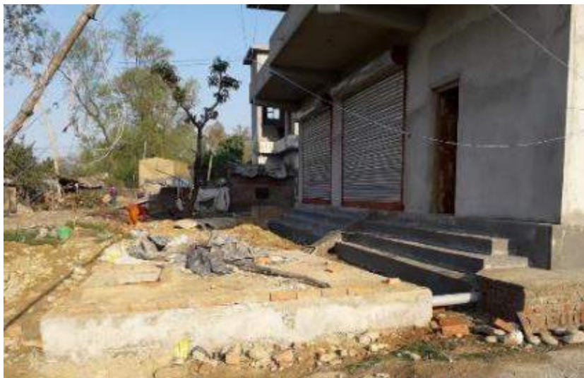
Figure 7: A fully lined tank under construction.
