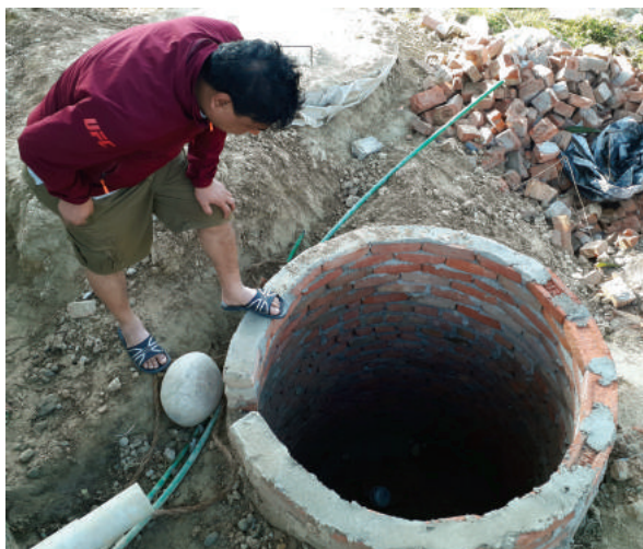
Figure 8 : A soak pit constructed to discharge effluents.
