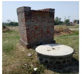
Figure 4: A concrete ring pit
