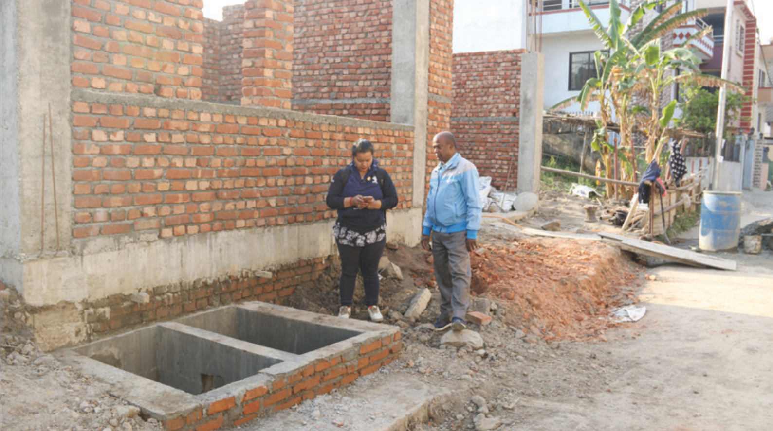
Monitoring of septic tank construction in field
