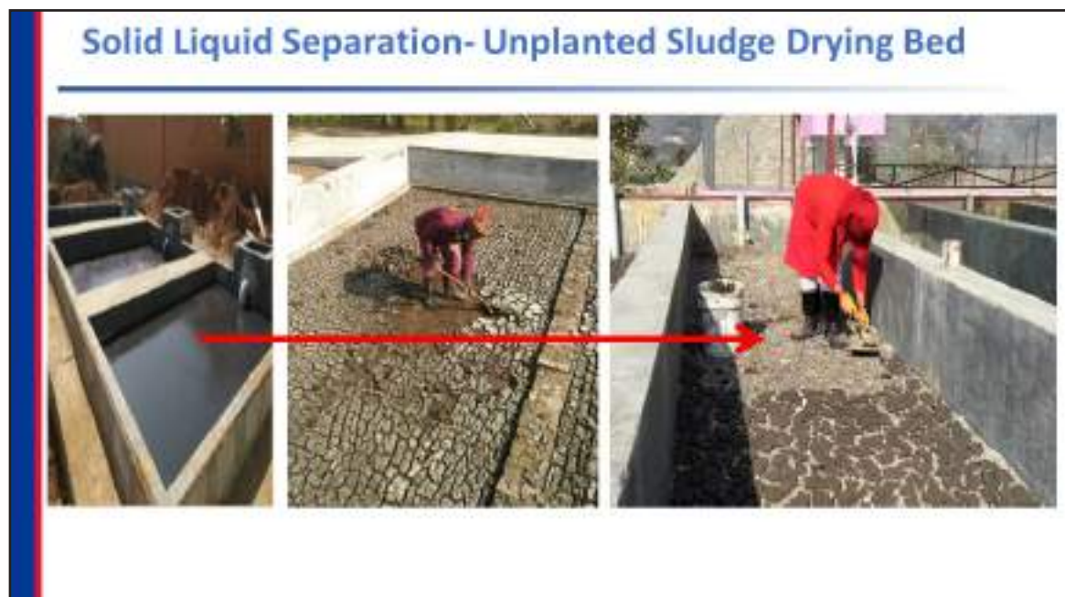
Example of the unplanted sludge drying bed
