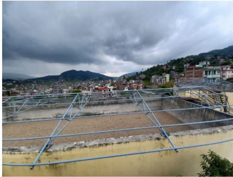
Figure 14: Overview of slow sand filter unit in water supply system developed under KVIWSP.
