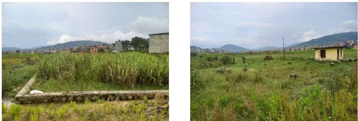
Figure 5: Overview of non-functional WWTPs in Budole and pumping station without pumping set.
