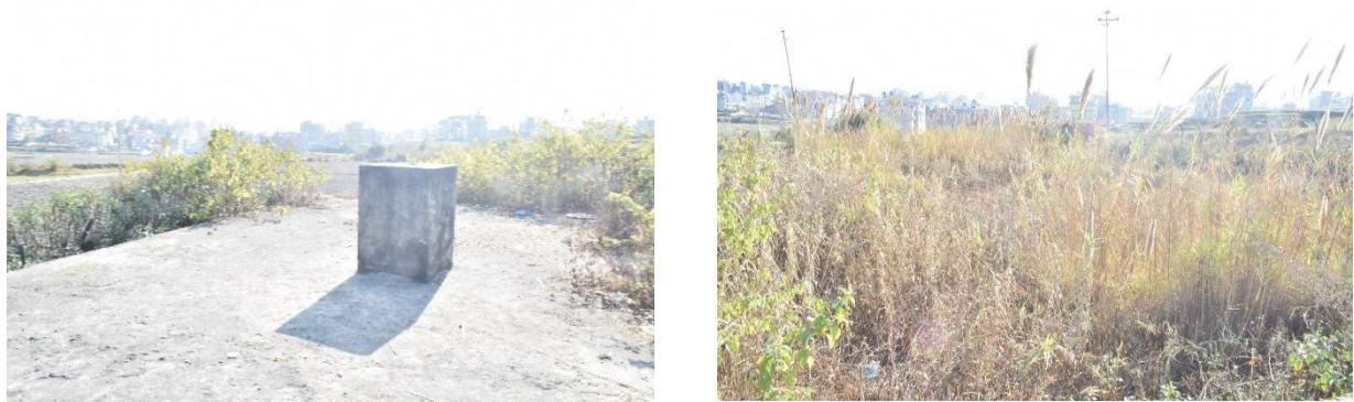
Figure 4: A deserted settler, untrimmed and overgrown reeds in the constructed wetland in Chandeshwori WWTP.
