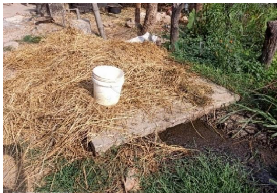
Figure 4: Toilet connected to Biogas digester.
