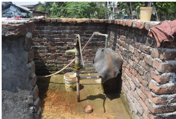
Figure 24: Handpump at surveyed household used for drinking water.
