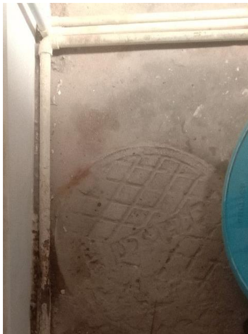
Figure 8: Top view of a fully lined tank in Birgunj.
