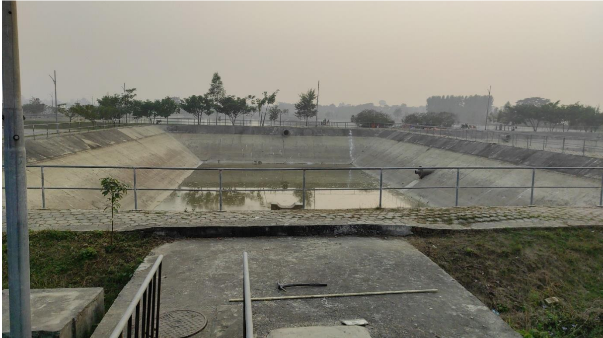
Wastewater Treatment Plant located in Birgunj.
