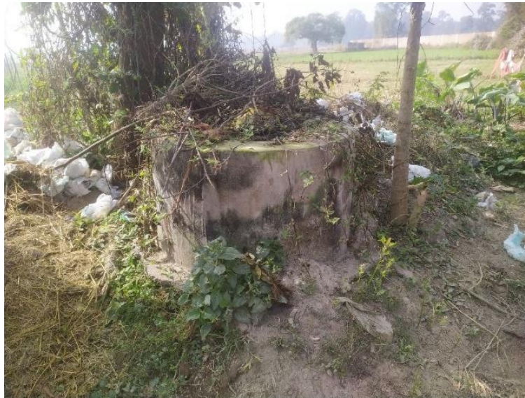
Figure 9: Biogas Digester in a household of Birgunj Metropolitan City.
