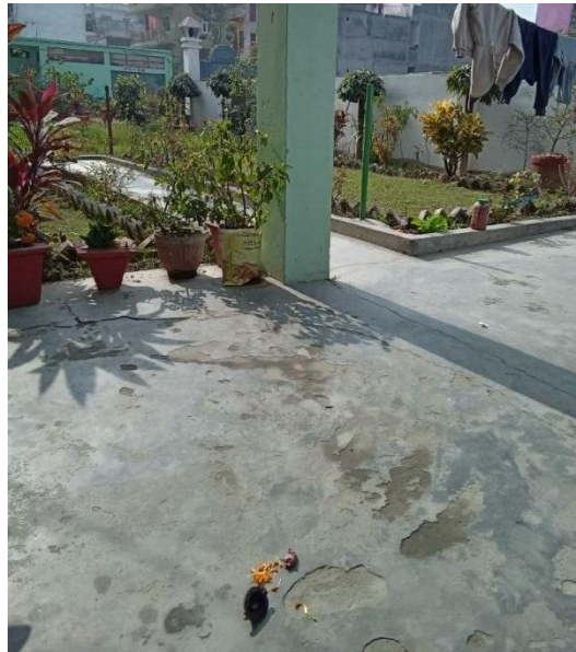
Figure 7: Top view of a septic tank in a household of Birgunj.
