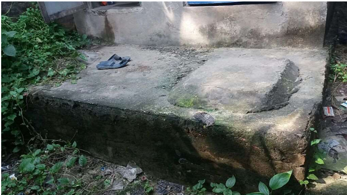
Figure 5: Containment with plinth level raised above ground to prevent inflow of runoff.
