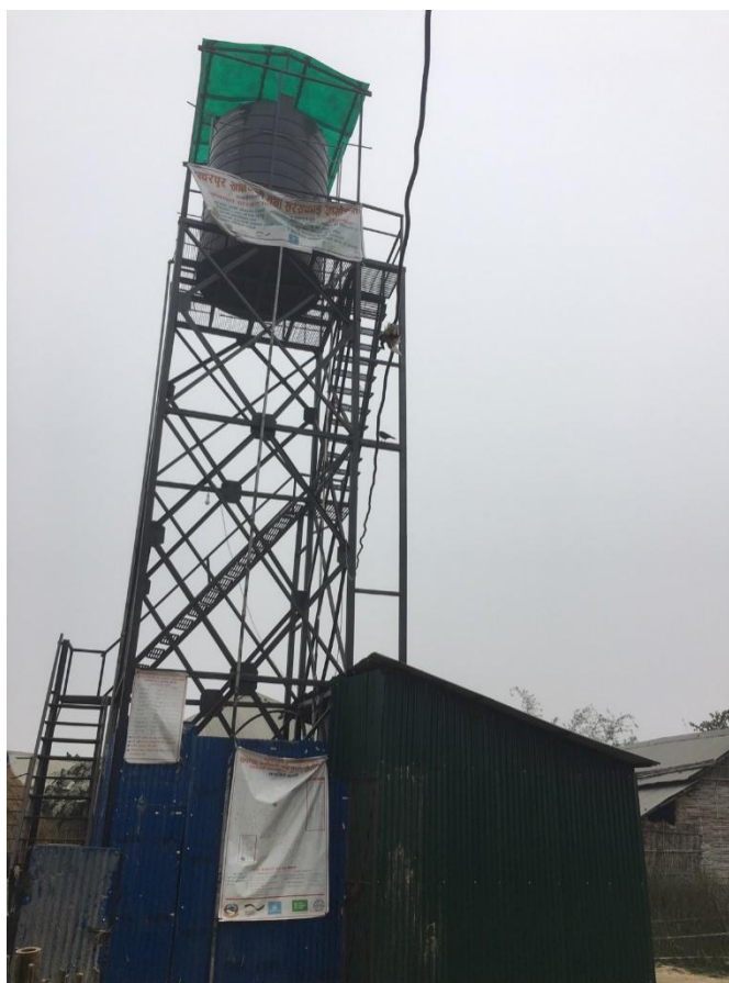
Figure 10: Overhead tank of Sundarpur Water Supply Scheme.
