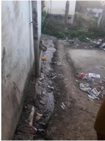
Figure 9: Overflowed faecal sludge from containment in the public toilet located opposite to Irrigation Office.
