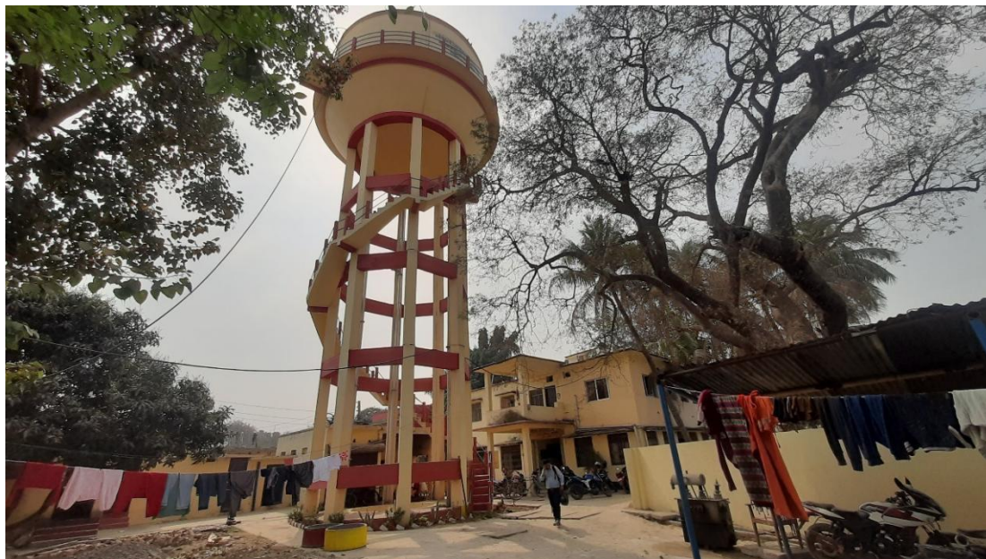
Figure 13: An overhead tank for distribution of water from NWSC Gaur Branch Office.
