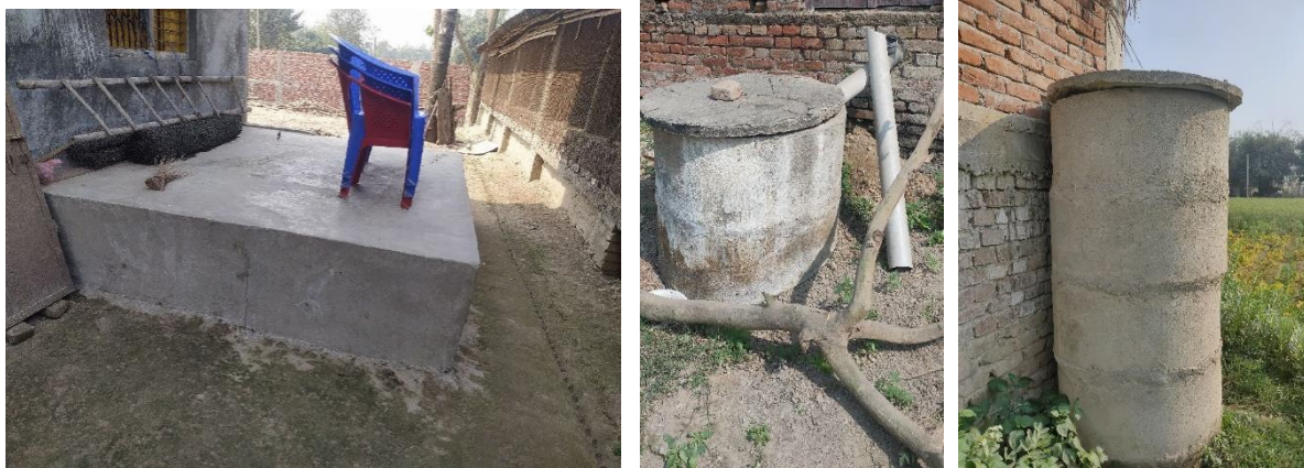
Figure 5: Containment with plinth level raised above ground to prevent inflow of runoff.
