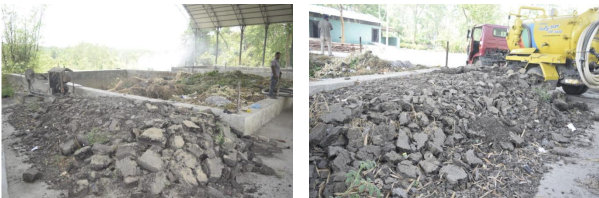
Figure 16: Manure made from human faecal sludge as seen in treatment plant.
