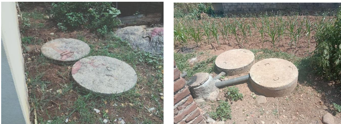
Figure 4: Inappropriate design of a twin pit.
