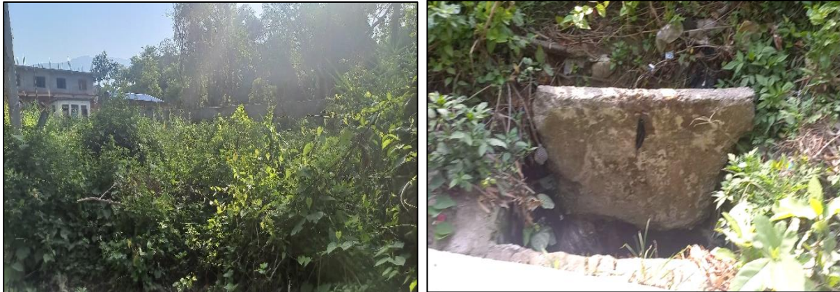
Figure 14: Status of wastewater treatment plant at Ward 10.
