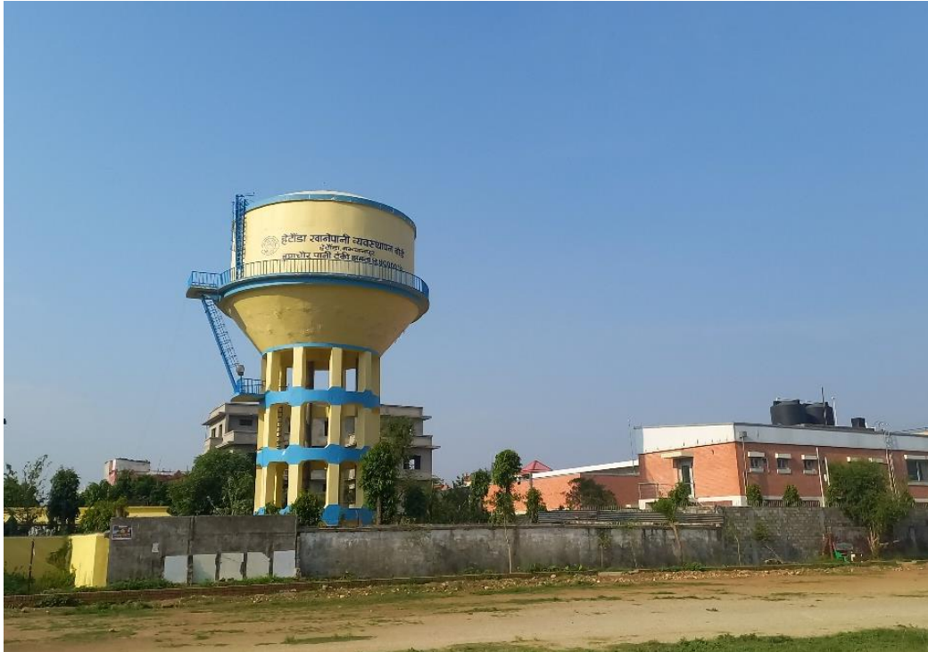
Figure 17: Overhead water tank at Huprachaur.
