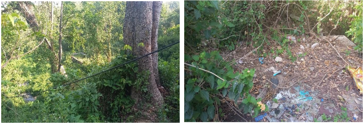
Figure 13: Status of wastewater treatment plant at Ward 10.
