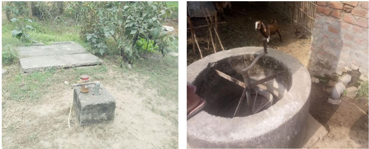
Figure 6: Types of biogas digesters in Kolhabi Municipality.
