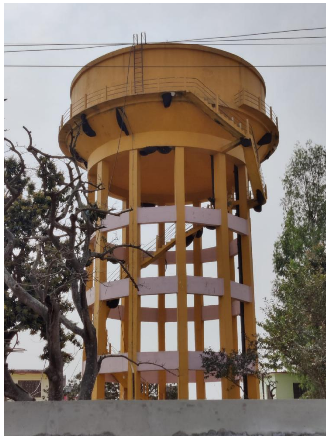
Figure 8: RVT operated by NWSC, Malangwa branch.
