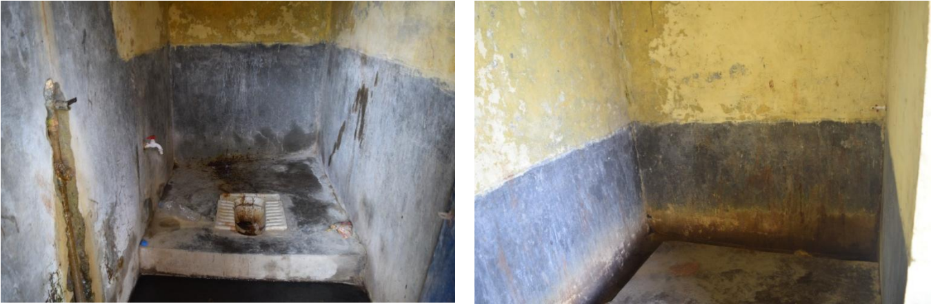
Figure 11: Status of pan (left) and urinals (right) of the public toilet at Mirchaiya bazar.
