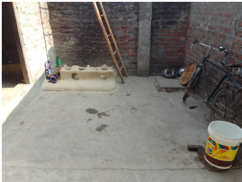
Figure 4: Top view of Septic tank in a household of Mithila Bihari Municipality.
