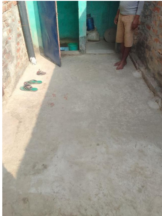
Figure 5: Top view of a fully lined tank in Mithila Bihari Municipality.
