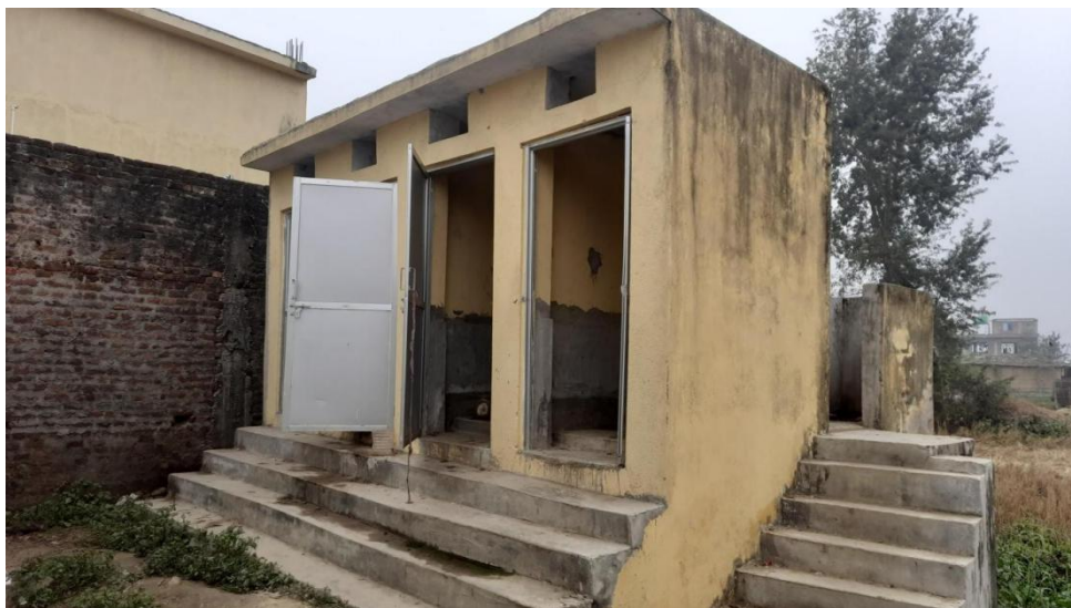
Figure 13: Public Toilet in local vegetable market area at Parsagadhi Municipality.
