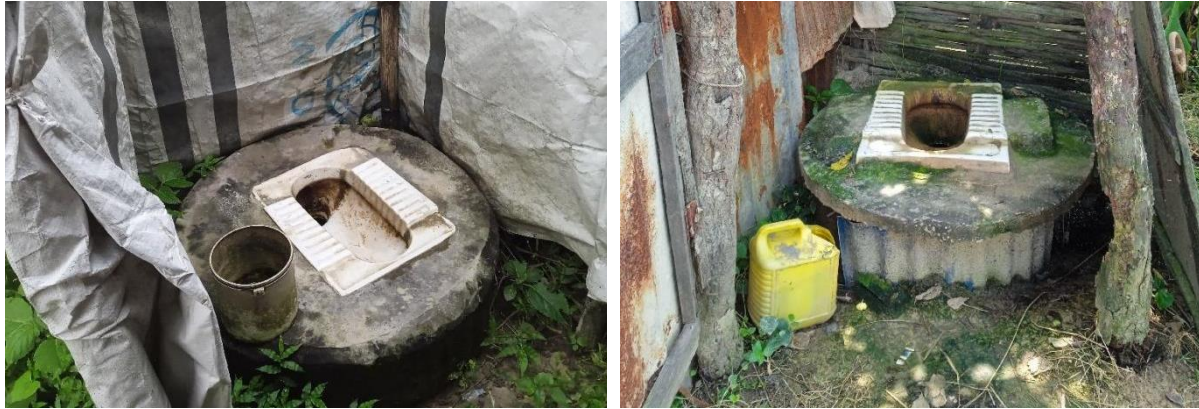
Figure 6: Types of unlined pits in the municipality.
