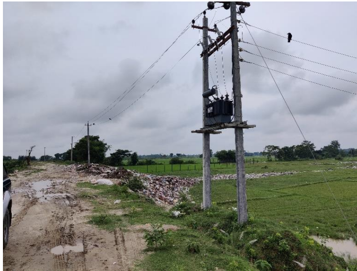
Figure 12: Solid waste dumping site at Khado, Rajbiraj.
