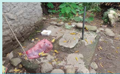
Unlined pit installed in sampled HH
