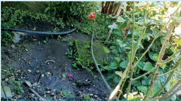
Unlined pit installed in sampled HH
