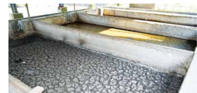
Gulariya faecal sludge treatment plant
