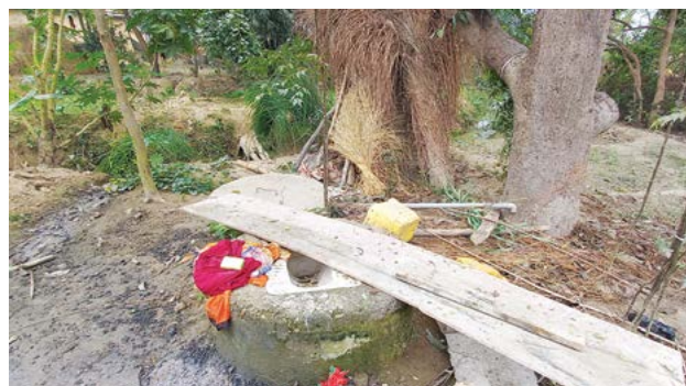
Toilet without superstructure which is not in use
