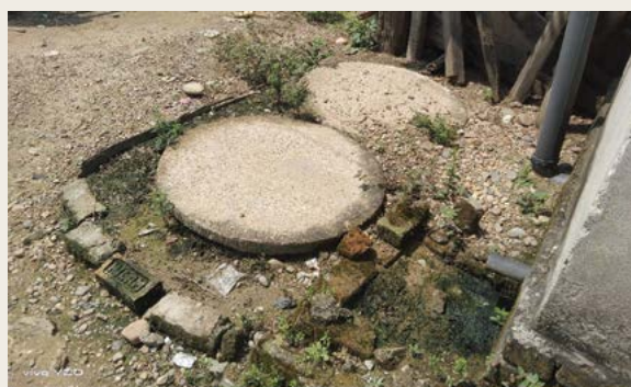
Twin pits installed in one of the surveyed household.
